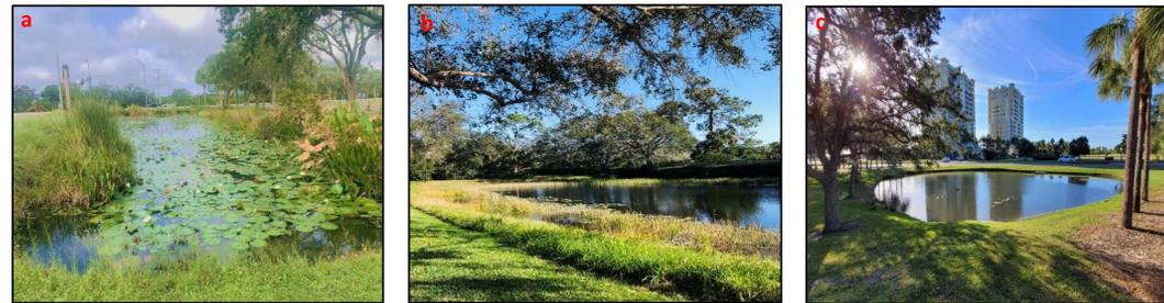
Figure 3: Three planting styles studied (a) stormwater ponds with planted banks and planted littoral zones., (b) stormwater ponds with no-mow buffer zones & planted littoral zones, and (c) conventional stormwater ponds with only turfgrass banks
