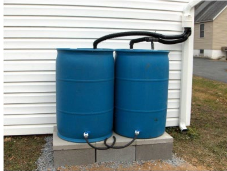
Figure 1. Rain barrel installation collecting from gutters. Credit: Kimberly Moore, UF/IFAS
