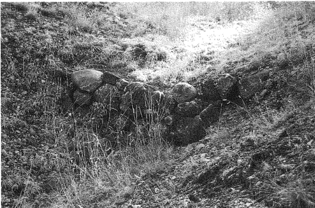
**Figure 4.** Water and soil control structure built by the Civilian Conservation Corps (CCC) in the 1930s near Mogollon, New Mexico. In addition to the multiple course construction, note (1) the uniformity in the sizes of the rocks, (2) the stacking of materials that involved a certain amount of deliberation, (3) the dipped elevation, (4) the way in which rocks were stacked in the channel, abutting the banks, (5) the lack of breaching, and (6) the sediment accumulation behind the structure.
