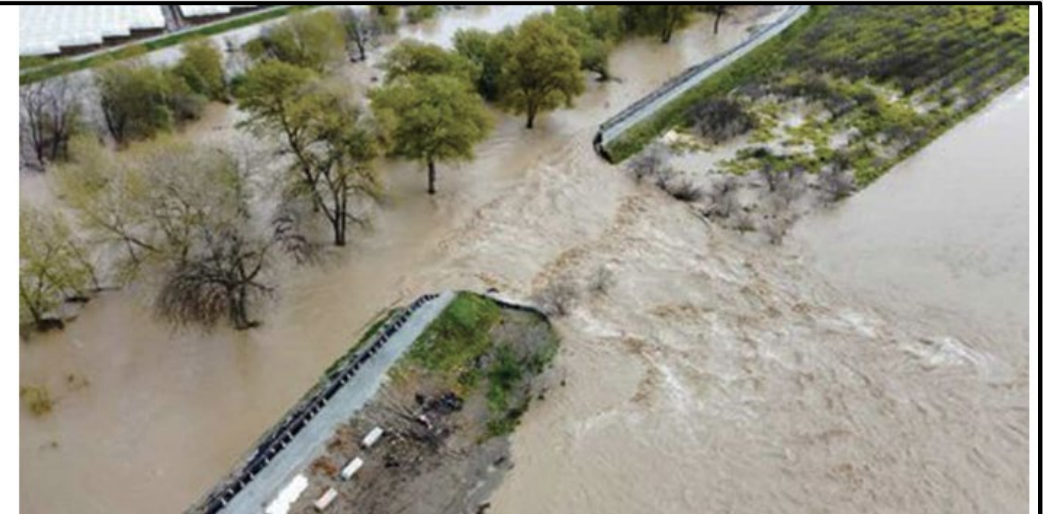
This drone image shows where the Pajaro River levee breached near Murphy Crossing Road. Photo: Alfredo Torres
