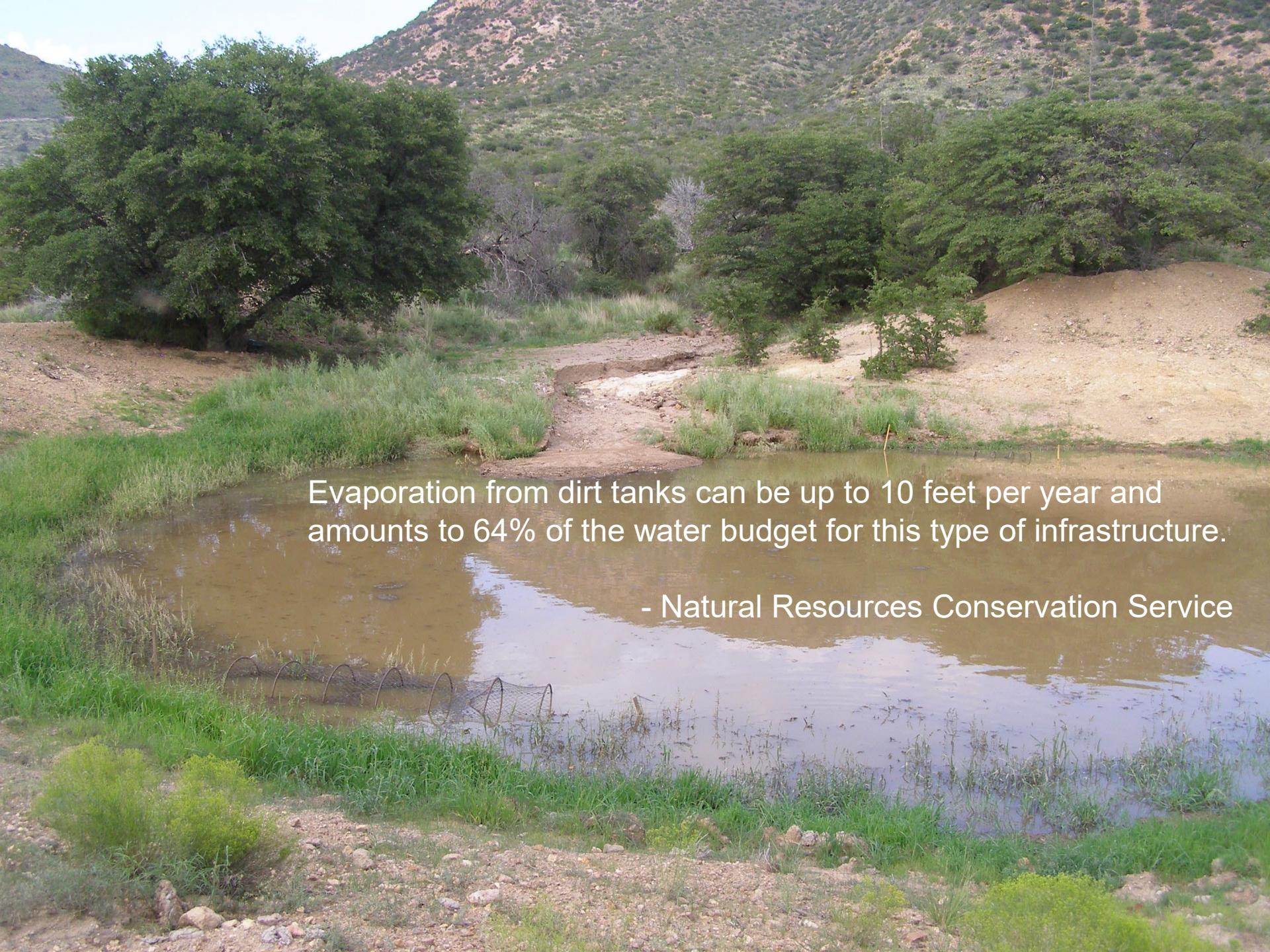
Evaporation from dirt tanks can be up to 10 feet per year and amounts to 64% of the water budget for this type of infrastructure.
