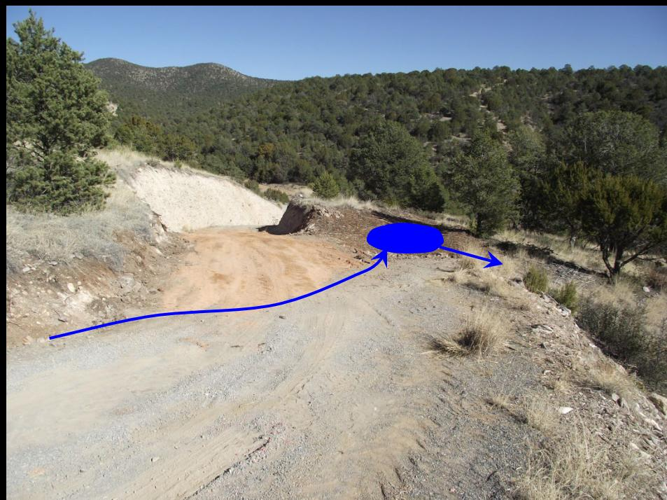
Problem: a rutted road captures hill slope runoff, eroding the road surface on the steep hill below, while increasing sediment and flooding in the arroyo.
