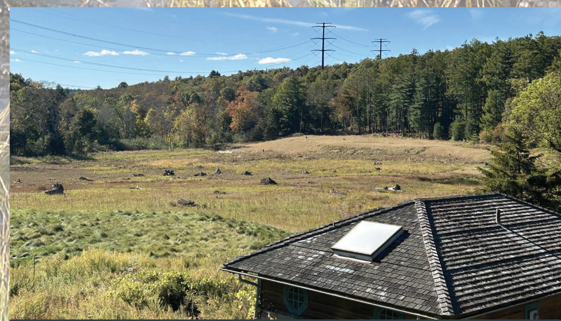
Pond 10 post restoration Wetland and stream overlook
