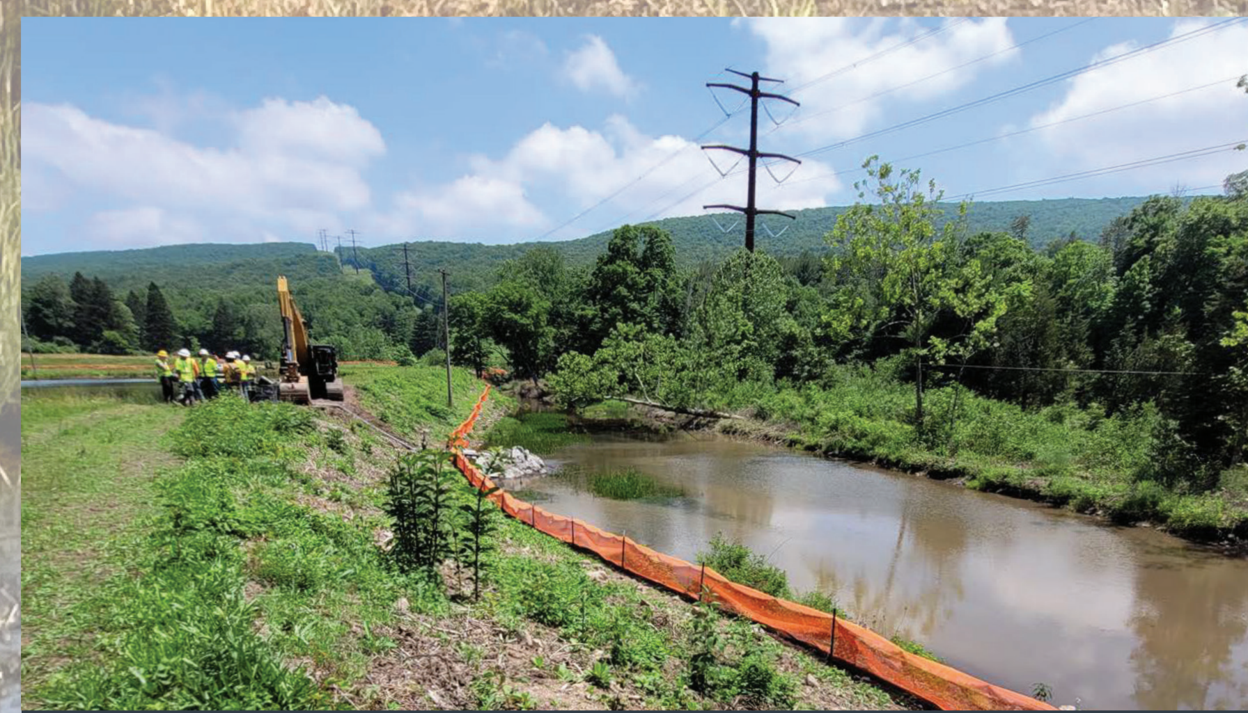
Van Campens Brook and Pond 10 (with dam) Pre-removal and floodplain
