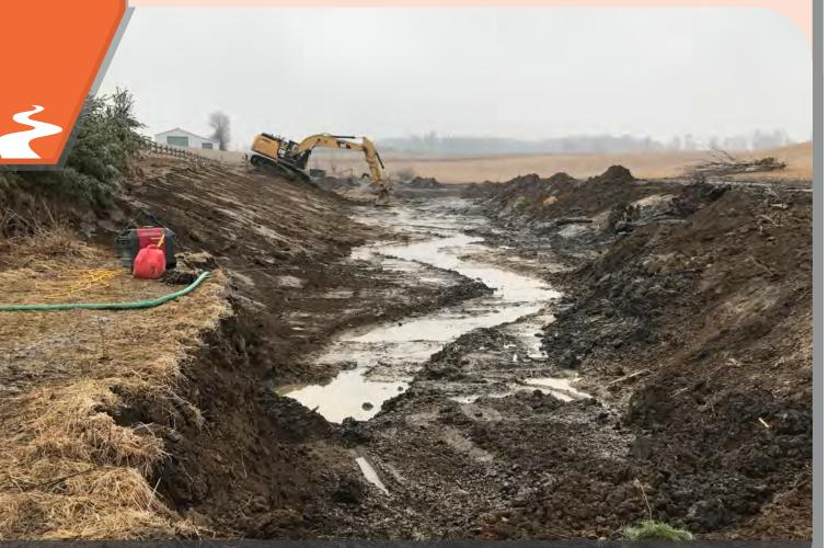
Construction in February/March 2017. New channel and wetland excavation. Water flows from pipe were pumped around the construction site
