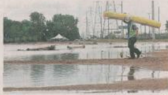
Erich Westergren of the Indiana Landscape Constructors holds a hay blanket to an island along the Roxana Marsh in the Grand Calumet River that will reduce erosion and encourage vegetation growth. Officials held a ceremony Monday marking the final stages of the Grand Calumet dredging and restoration project.
