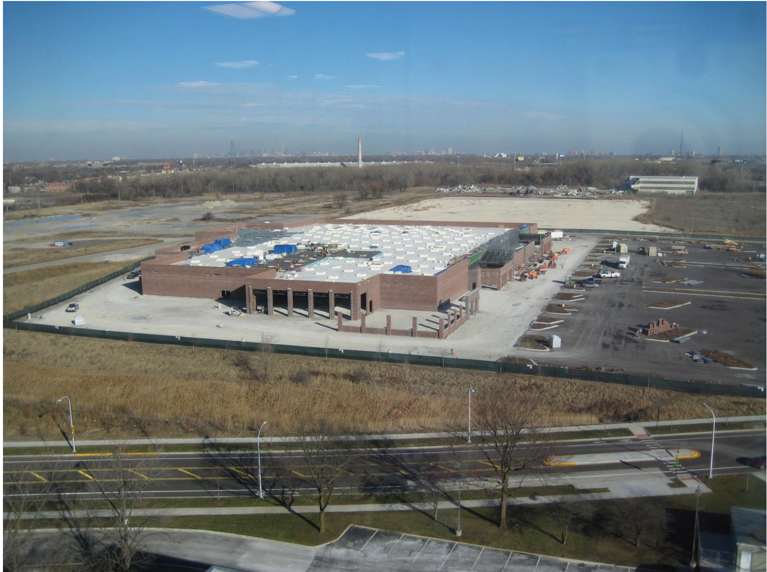
Ariel View Construction
