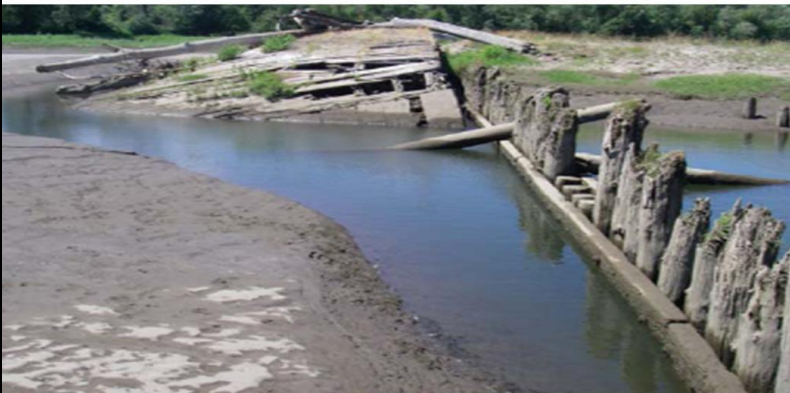
Transverse Pile Dike
