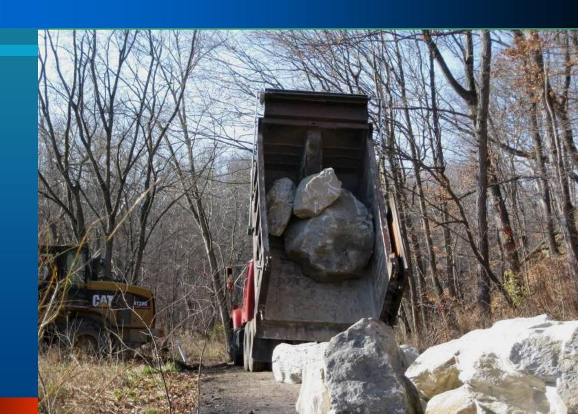
R-5 & R-6 stone on left (used for key & to choke larger stone), large riprap on right used for Engineered Rocked Riffles (ERR), Single Stone Bendway Weirs (SSBW), & bank stabilization.
