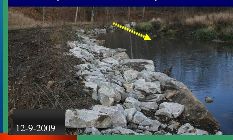
RAIN & HIGHER FLOW-Looking @ a right bank repair. Deep but Bendway Weirs are working well.
