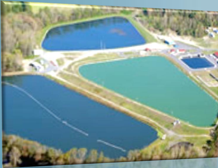
Laurel Wastewater Treatment Plant Upgrade - 2007
