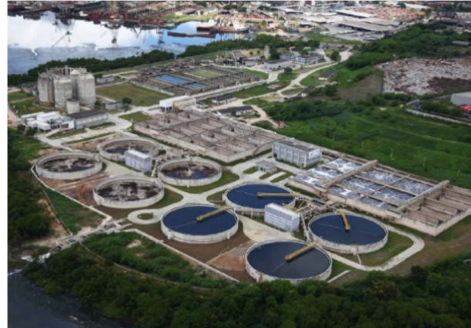
Alegria Waste Water Treatment Plant
