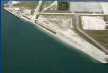
Aerial view of the start of the project.
