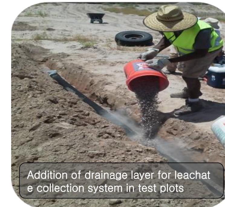
Installation of leachate collection pipes in test plots
