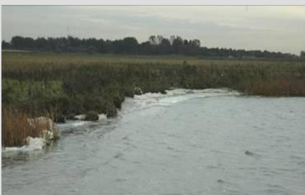
IJsselmeer foreshore nourishment
