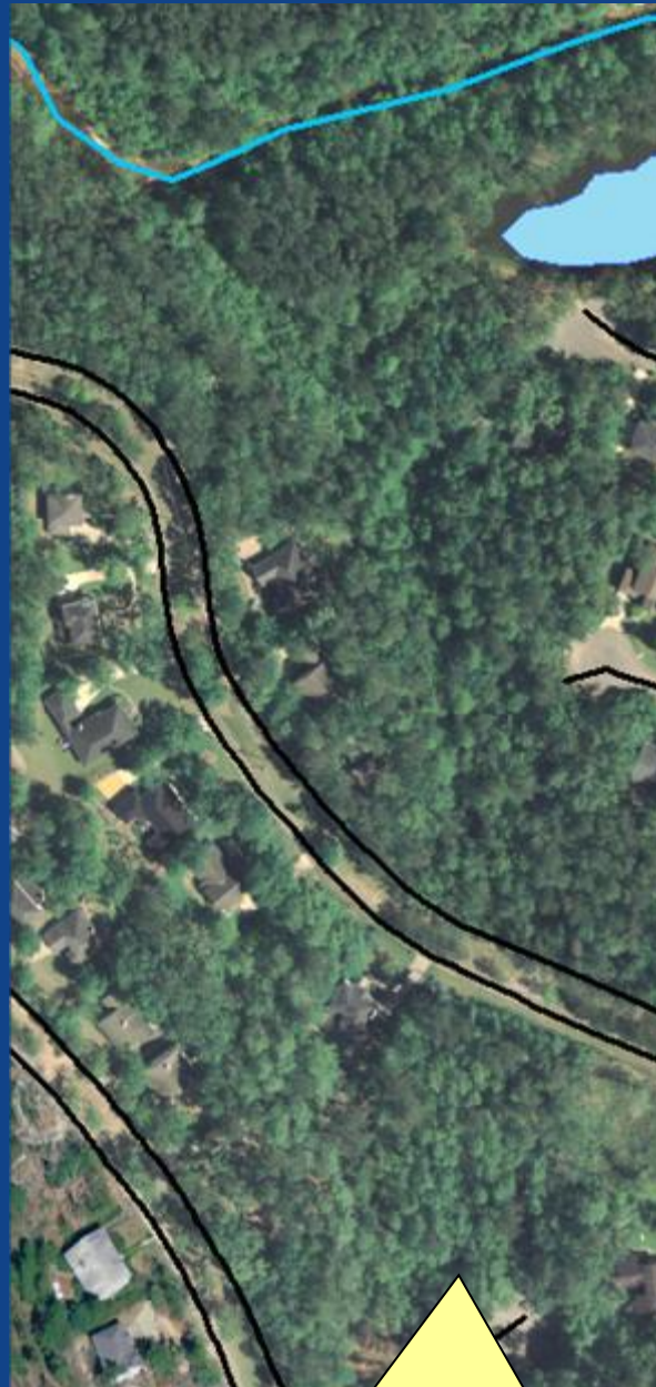
Gully with Headcut ?
