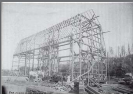
Framing a barn, 1907.
