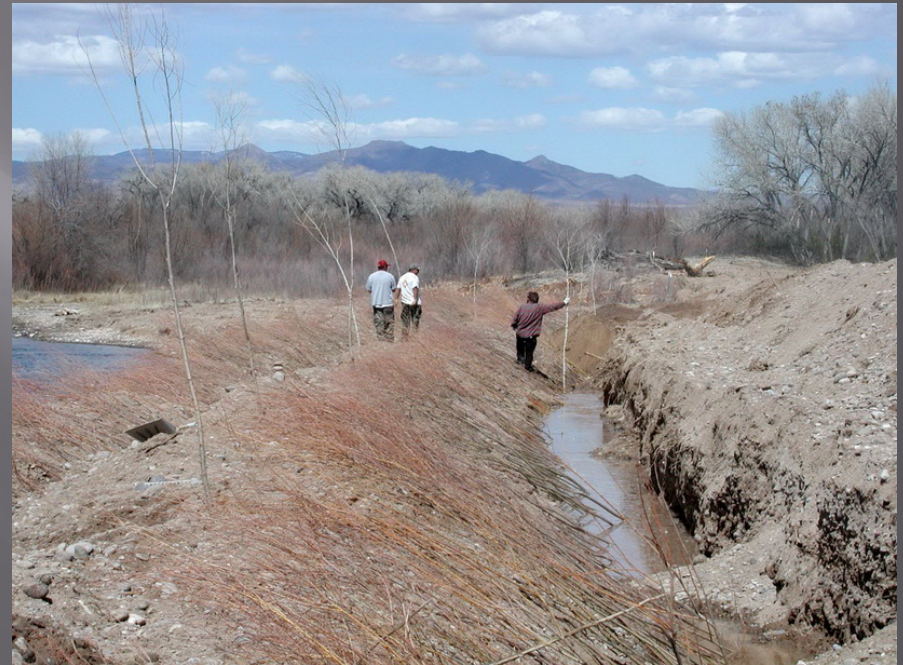
Willow swale construction
