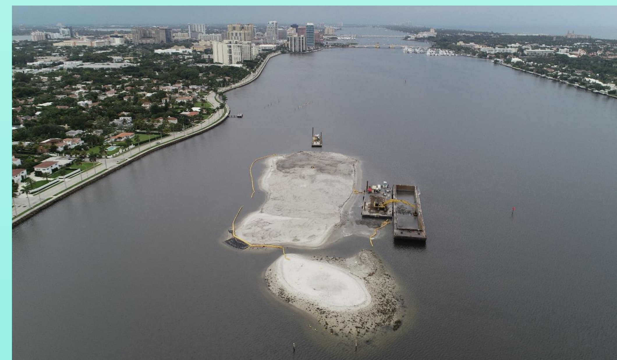
Figure 4: Aerial provided by Taylor Engineering May 2019 of ICWW material being placed at Tarpon Cove
