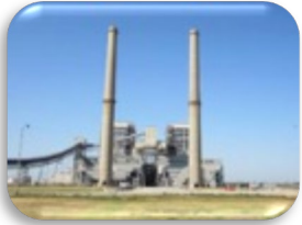
Oklahoma Gas & Electric Power Plant
