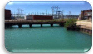
NRG Power Plant
