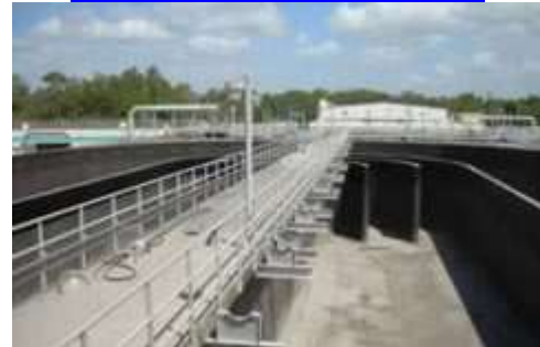
Eastern Water Reclamation Facility
