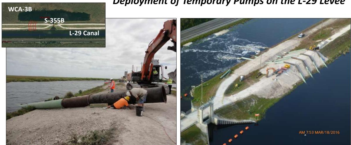
Deployment of Temporary Pumps on the L-29 Levee
