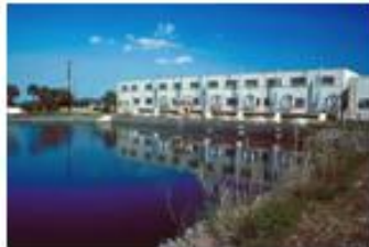
Reservoir pump station
