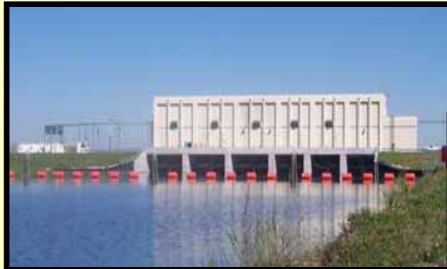
Water Management Operations
