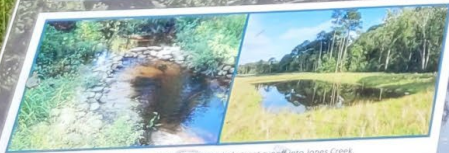
Rock vanes (left) and stormwater ponds (right) used to help treat runoff into Jones Creek.
