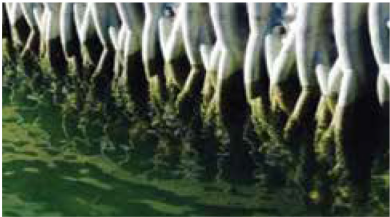
Example of seawall texturing showing contributor Dr. Keith Van de Riet's Mangrove Reef Wall System.
