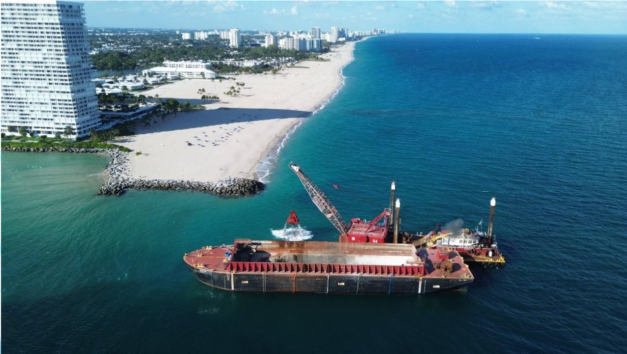
Photo: Foth Infrastructure & Environment
