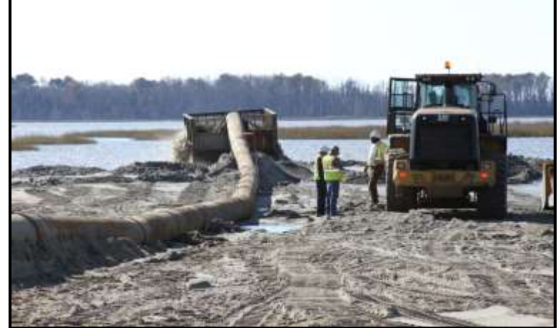
Sand Pumping to Close Breaches (Tim Boyle, USACE)
