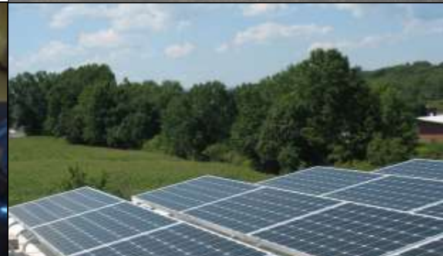
Solar Panel Installation (Photos: USFWS)
