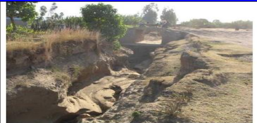
Gullying from poor drainage control
