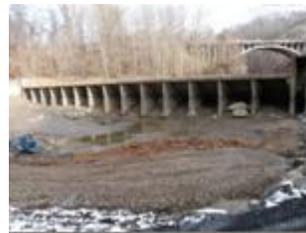
The former site of the Simkins and Union Dams will also be visited. Union Dam was removed from Oct 2009 – Sept 2010 using a heavily engineered approach with multiple river diversions and realignment of the stream channel. In contrast, the Simkins Dam removal using a passive sediment management approach with release of approximately 80,000-
