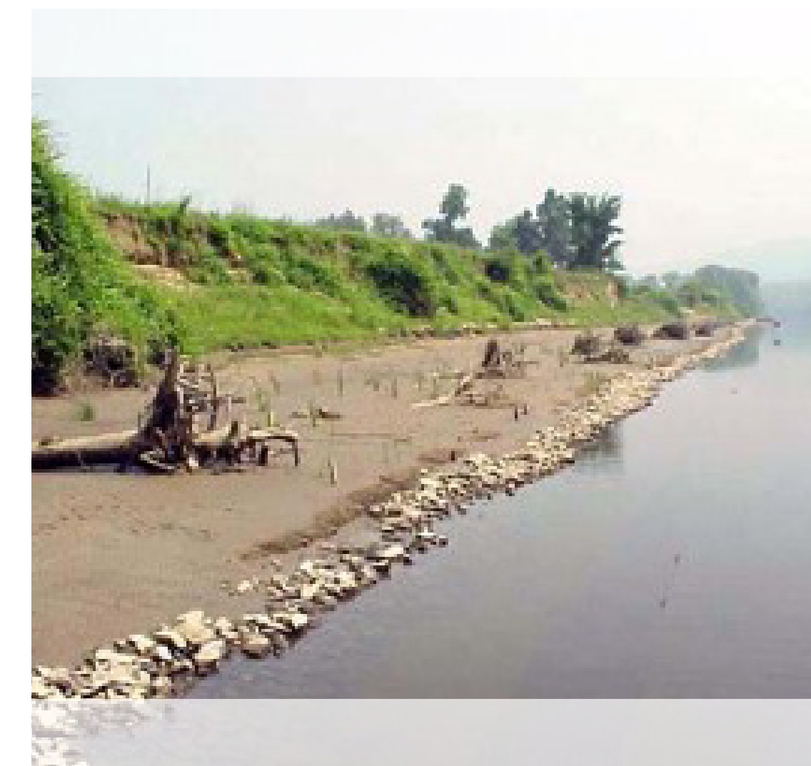
Building a new shoreline using stone, logs and plants - 1999
