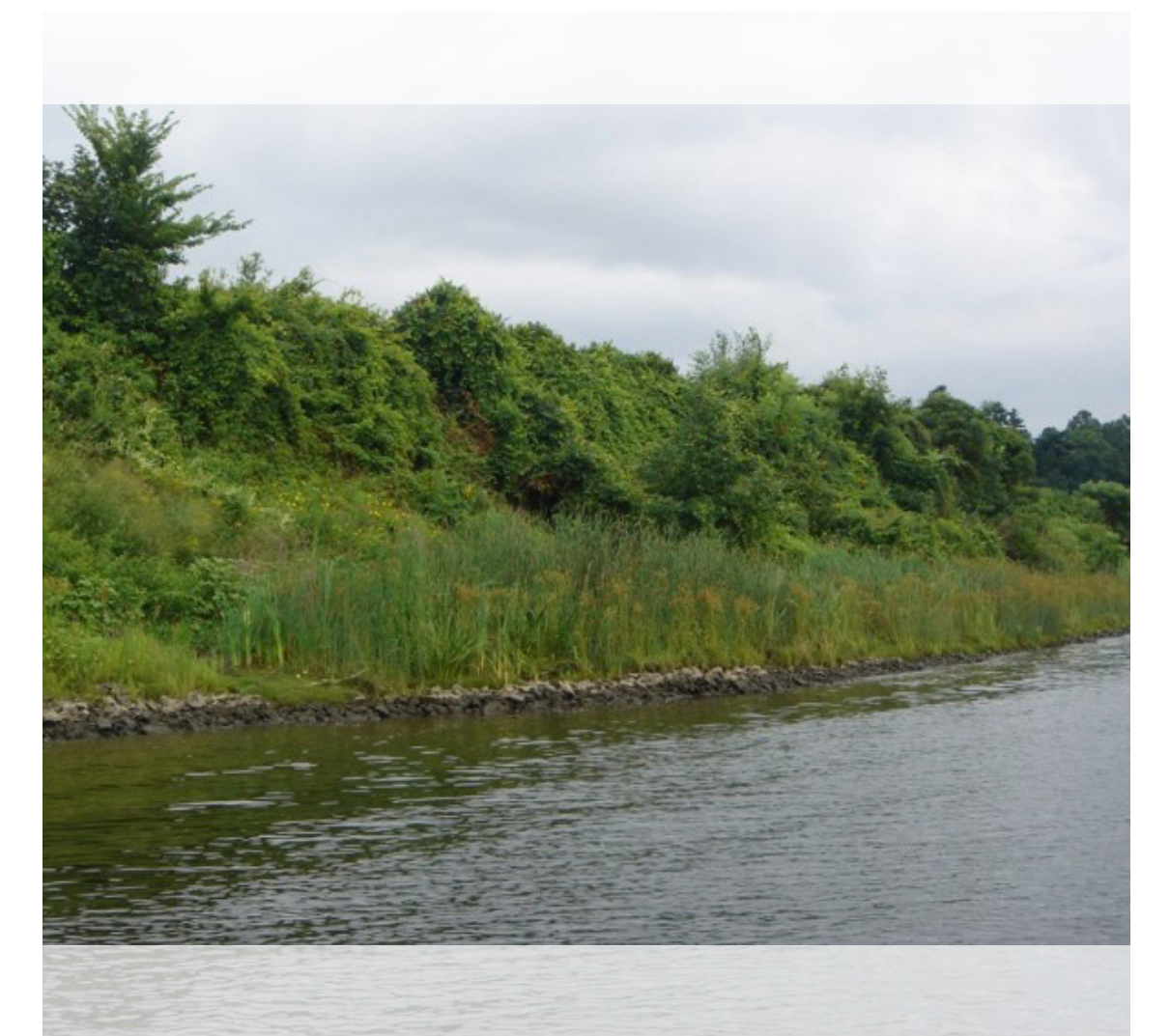
New shoreline - 2005 Post Construction
