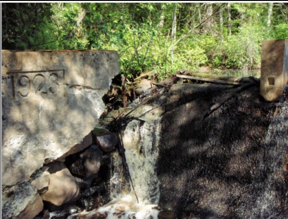
Right Spillway Abutment, Tack Factory Dam
