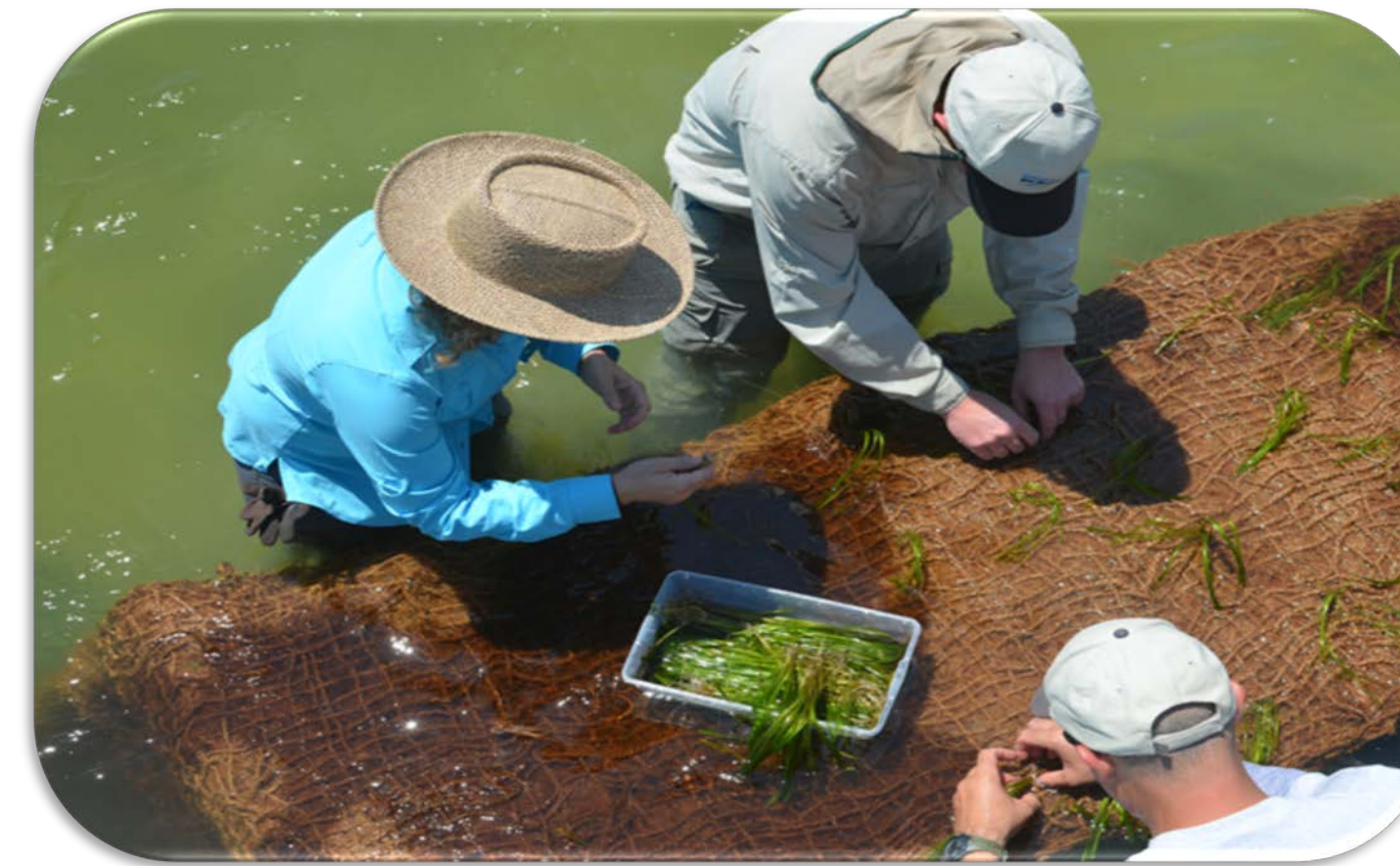
Eelgrass sod mats consisted of coconut coir fiber mats (15' x 3') planted on six inch centers with the 'Rockstar' variety of eelgrass ( Vallisneria americana ).
