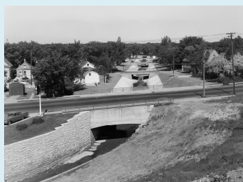
Figure 2. 1961 photograph of the recently lined KKR.
