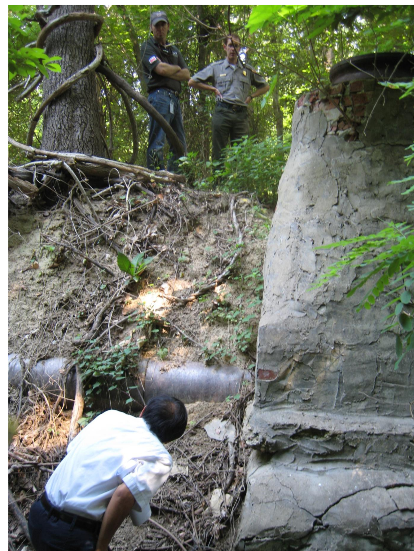
Figure 4. Officials examine the sewer line prior to restoration
