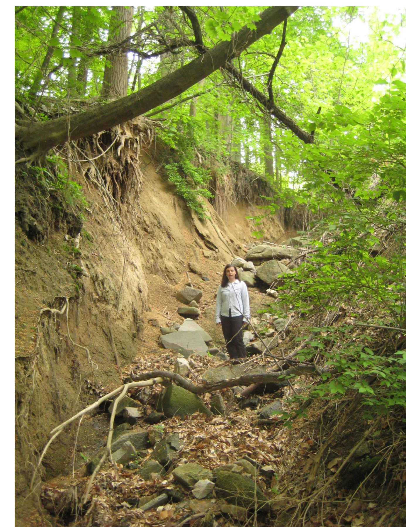
Figure 8. Erosion along Soapstone Run, a future RSC project
