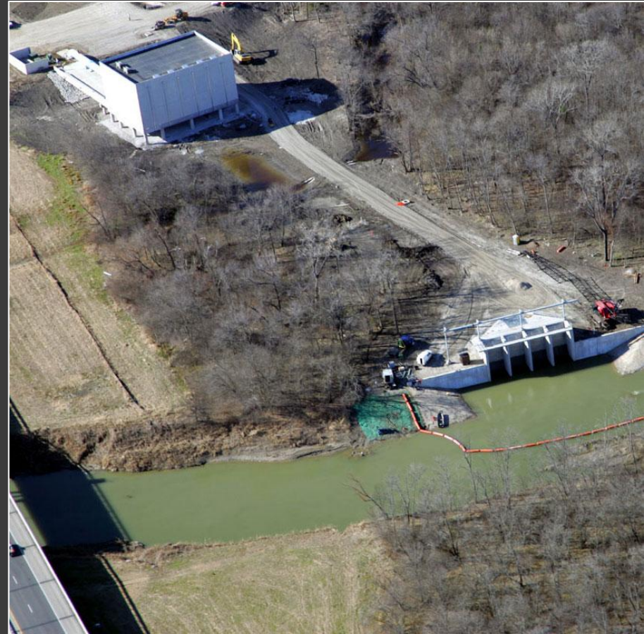
Trinity River Diversion Pump Station
