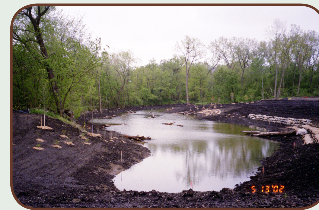
Channel restoration using bioengineering techniques
