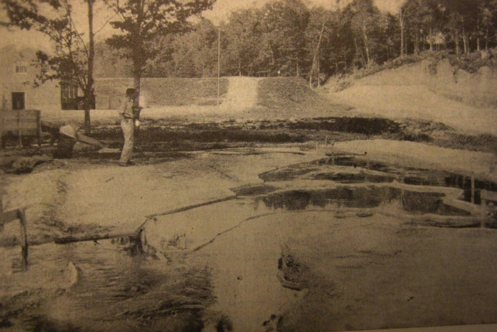
Model of Birds Point-New Madrid floodway under test
