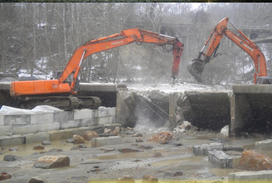
Diversion Channel (fabric lined) to Divert Water through Breached Dam
