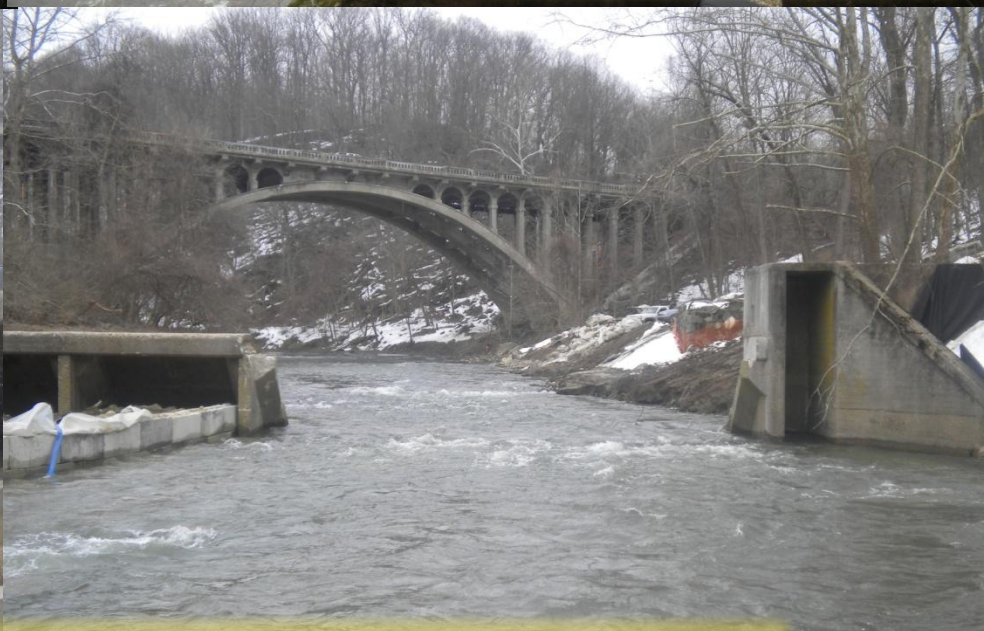
Diversion Channel (fabric lined) to Divert Water through Breached Dam
