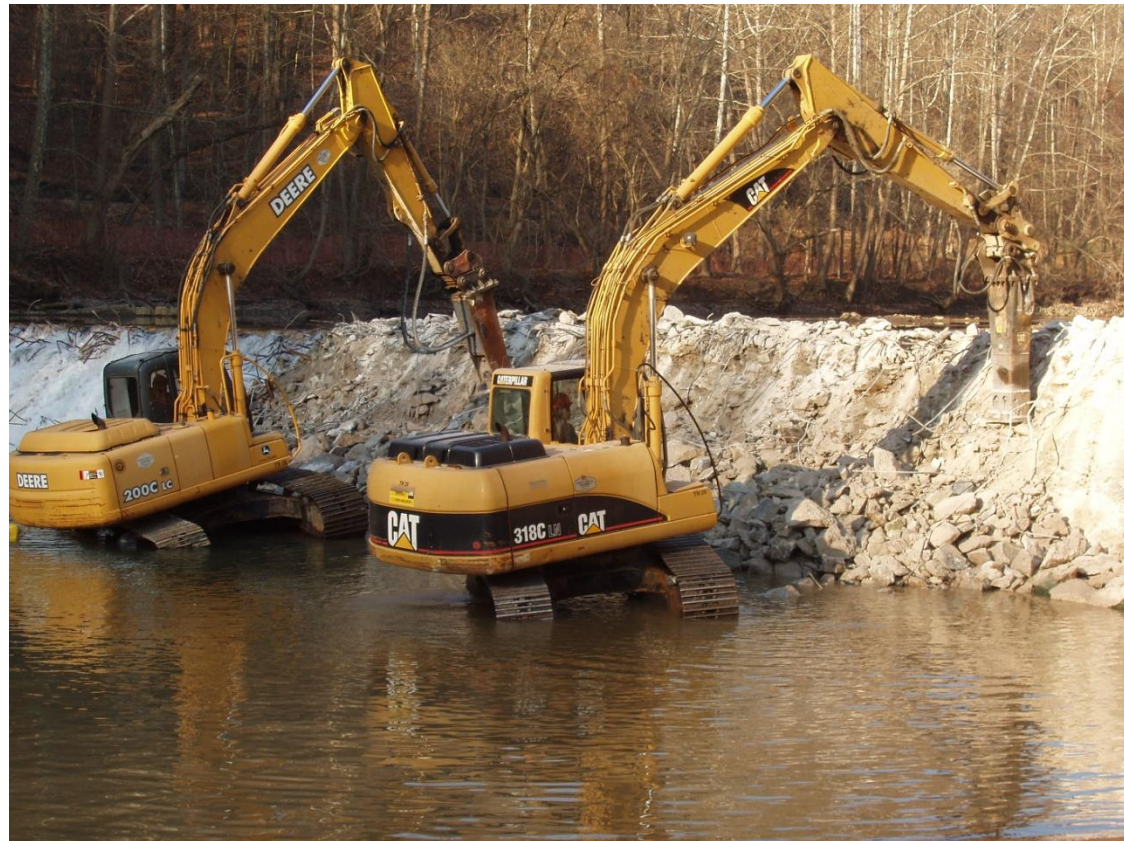
Simkins Dam Removal
