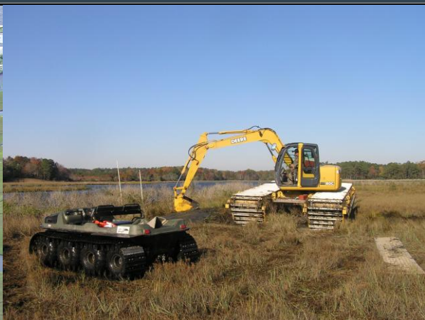
Installing Ditch Plugs
