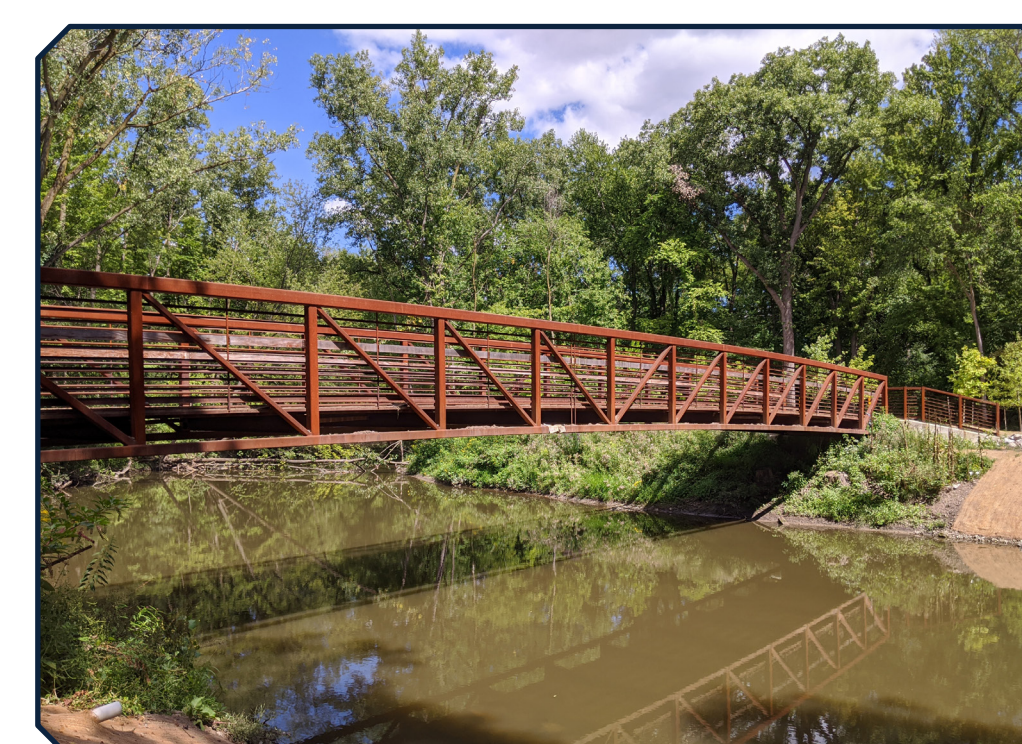
Maintenance & access bridge constructed.
