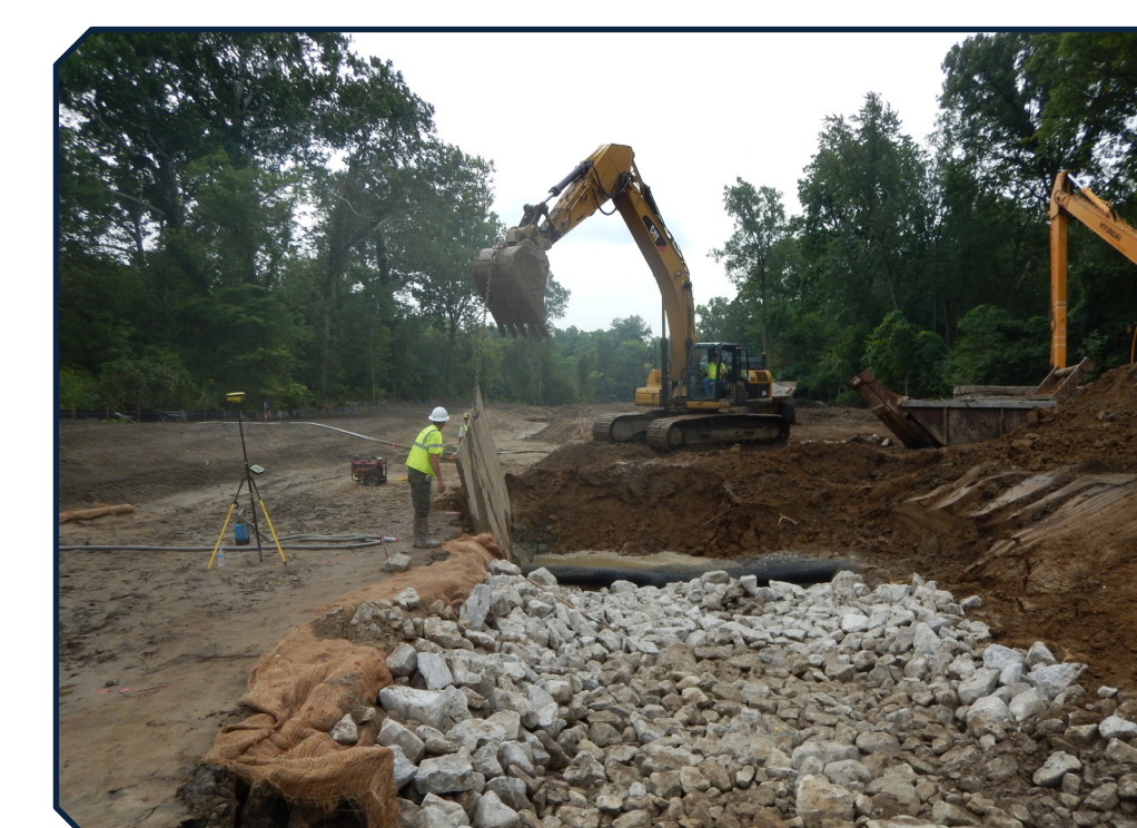
Construction of fishway.
