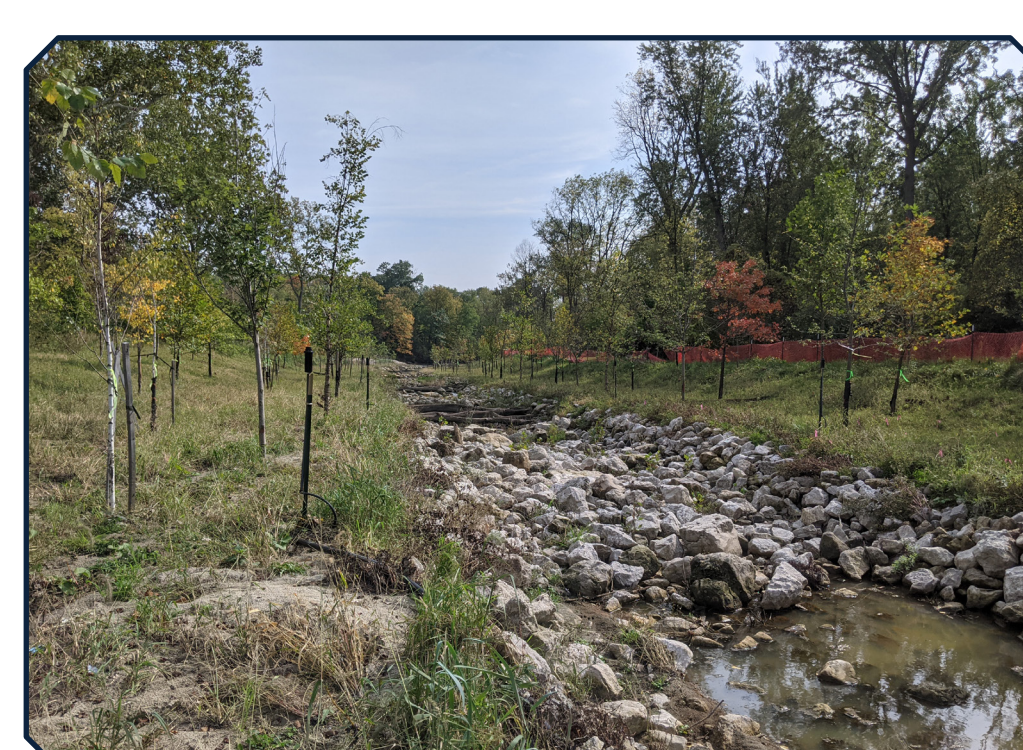
Establishment of vegetation important to stabilize the fishway.
