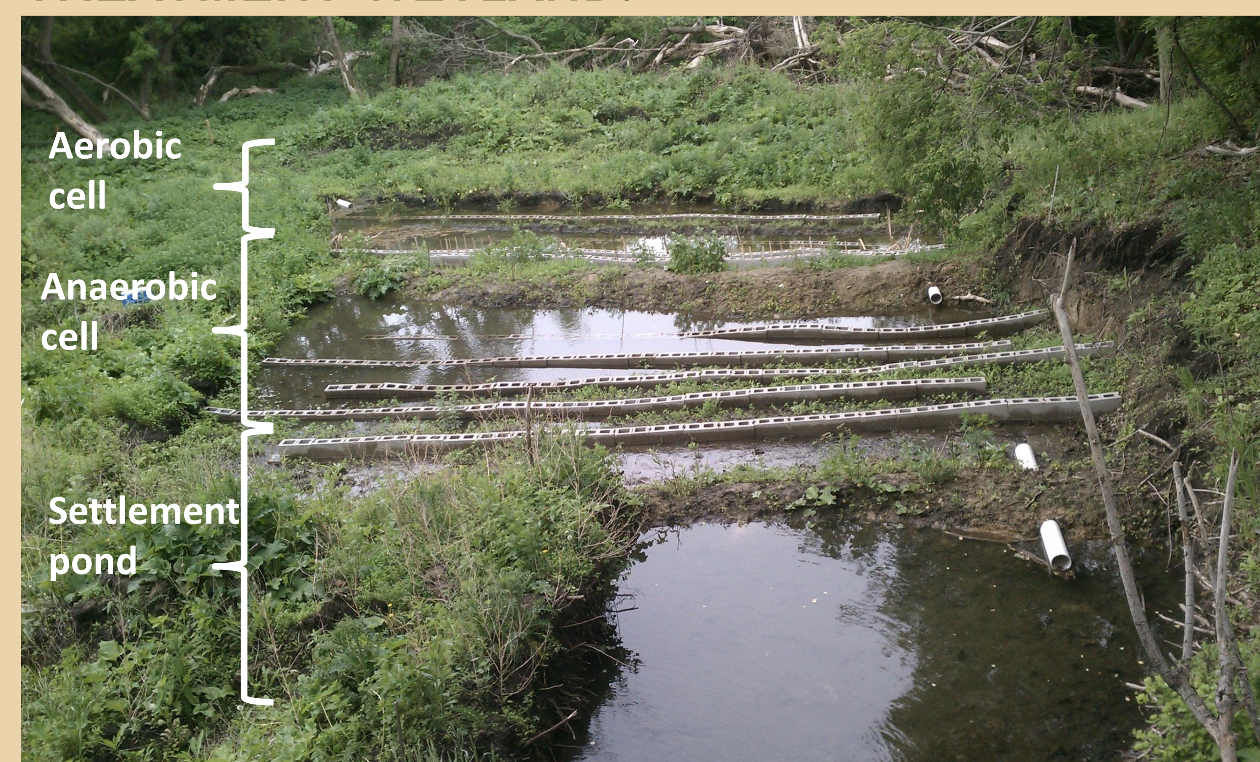
Fig. 1 TW with settlement pond and two treatment cells
