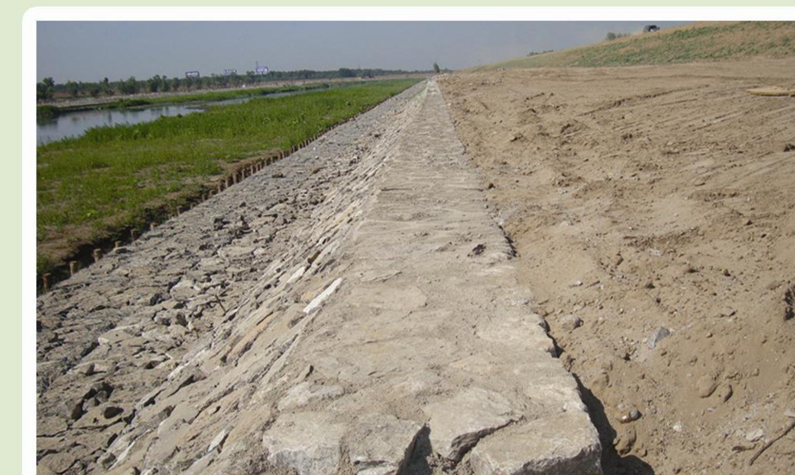
River bank stabilization
