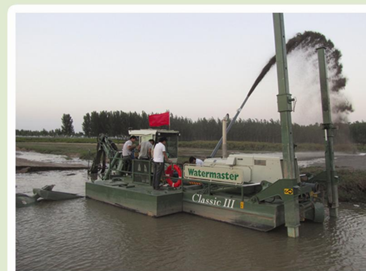
Dredging the river bed with the Multifunctional and Environmental Friendly Dredger
