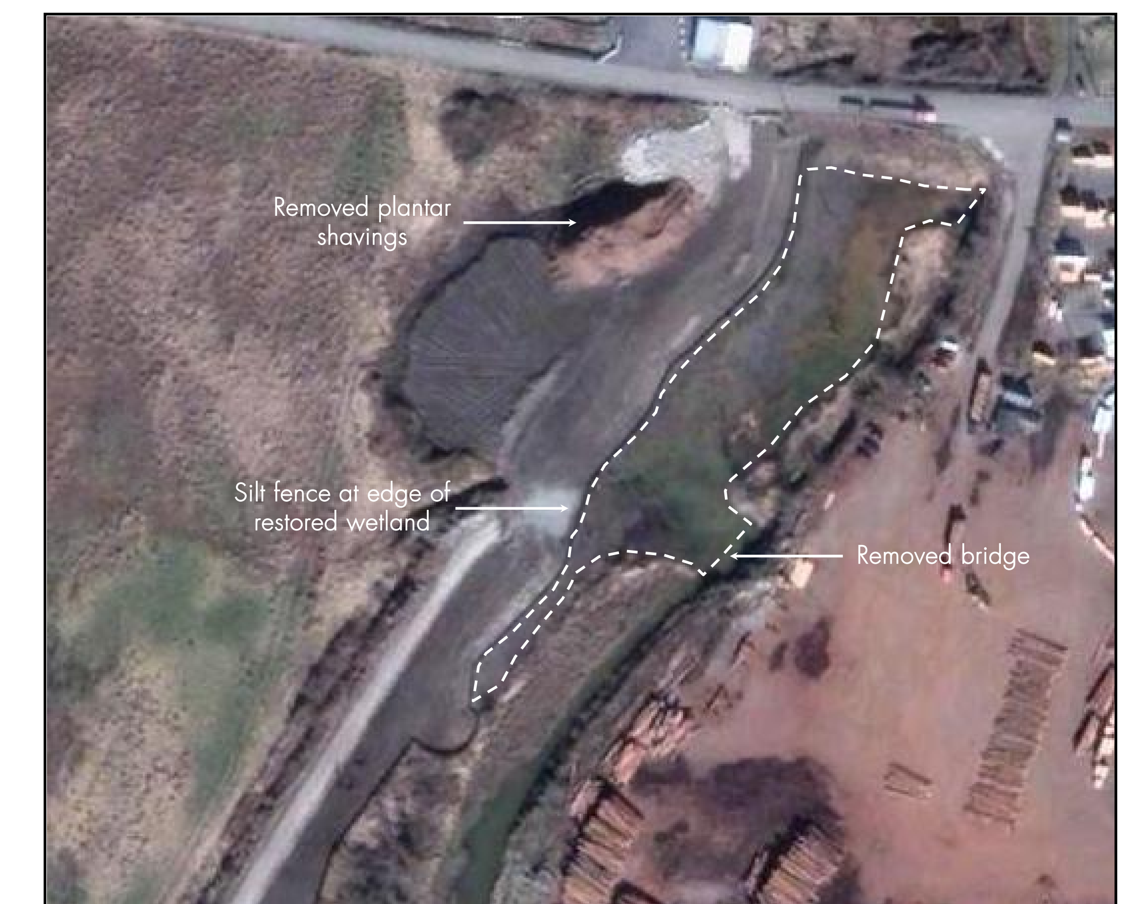
Figure 5. South parcel buffer enhancement and wetland restoration after completion of grading in 2005.
