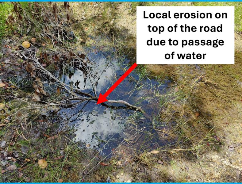
Local erosion on top of the road due to passage of water
