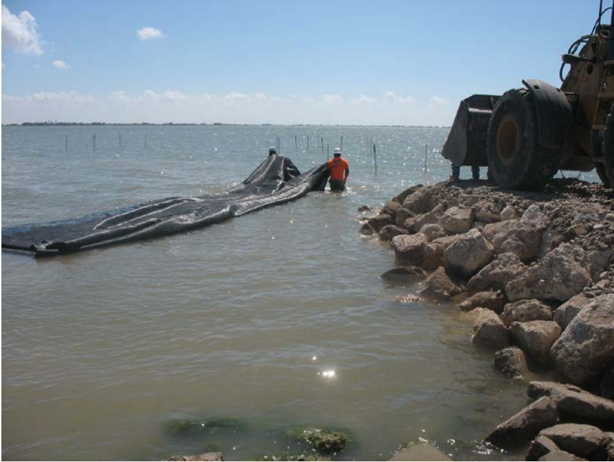
Geotextile Fabric Placement
