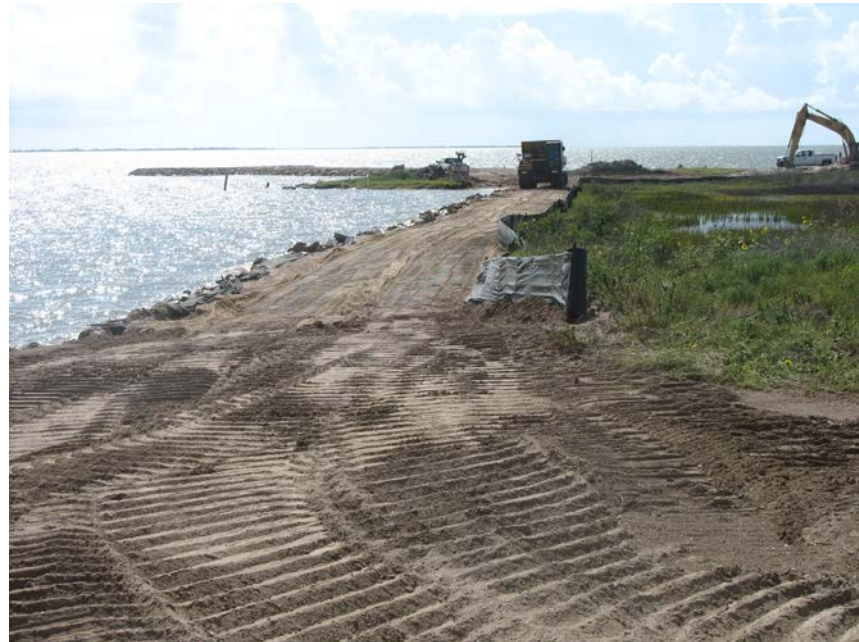
During Construction, North Beach
