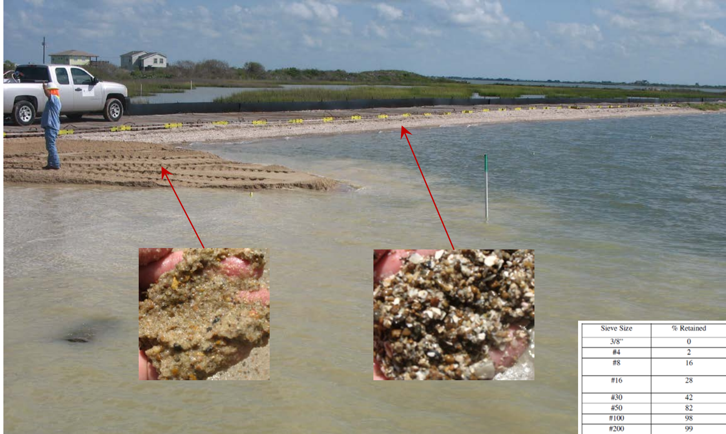
Equipment Access – Wood Pallet Road Along South Beach
